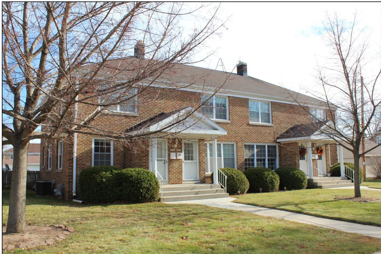
2717-2723 N. 12 th Street (1949) is one of the six, four-unit apartment buildings in the proposed Northern Apartments Historic District.
