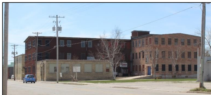
This complex of buildings, built between 1911 and 1924, functioned as the Sheboygan Fibre Furniture Company from 1913 to the 1940s, 2012-2024 N. 15 th Street.
