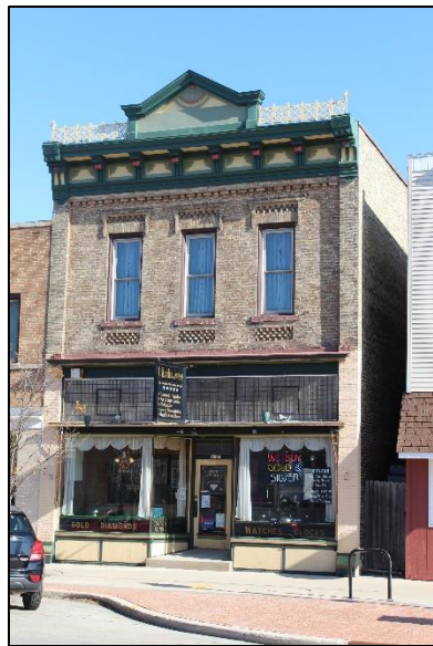
Hilmert Building (c1884), 1103 N. 8 th Street.
