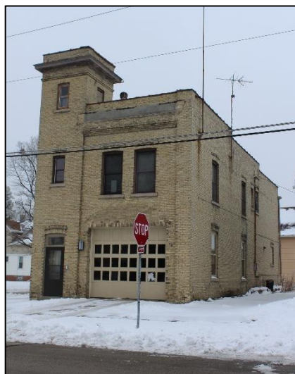
Hose Company No. 3 Fire Station (1904), 1827 N. 10 th Street.
