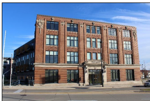
C. Reiss Coal Company Office Building (1912; 1961; 2007), 1011 S. 8 th Street.
