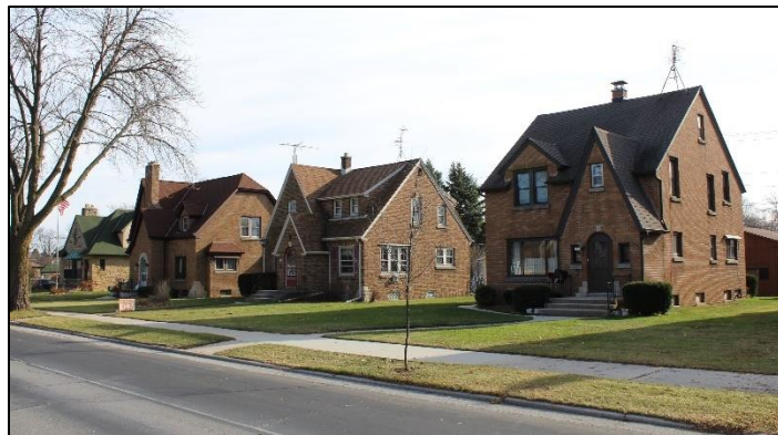
1103, 1107, 1113 and 1119 North Avenue (l to r) in the proposed North Avenue Historic District.
