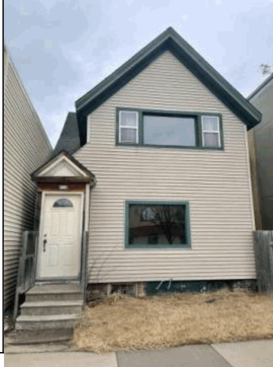
1 SF; building assessed value is $63,000
