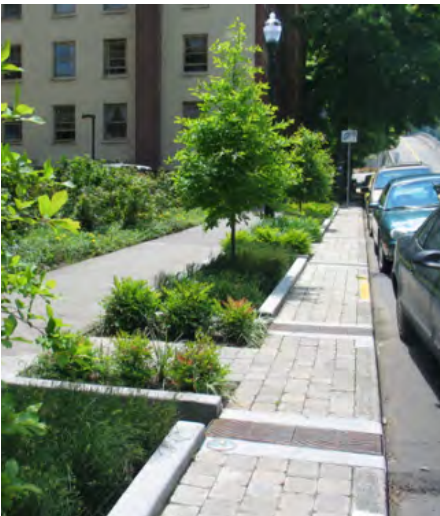
Parking adjacent to green infrastructure stormwater management Image source: GRAEF
