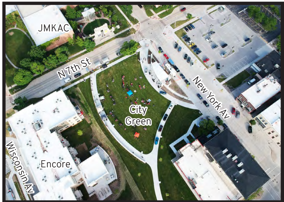
Aerial view of City Green. Three new pedestrian connections—at Wisconsin Avenue, mid-block through City Green, and at New York Avenue—were developed following the demolition of the former Boston Store building and subsequent development of the City Green and Encore apartment projects. Image source: City of Sheboygan.
