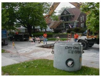
Precast Manhole with Rubber Boot
