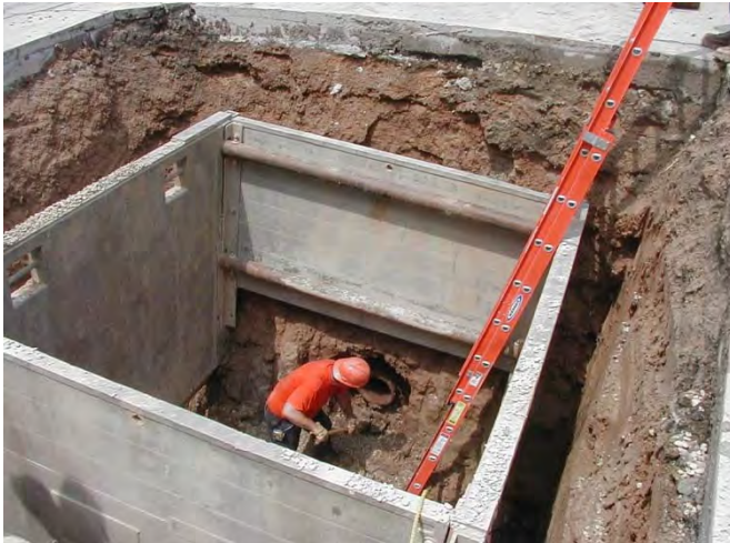
Preparing to Install a new Sanitary Manhole
