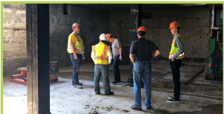
Basement Renovation in Progress at City Hall
