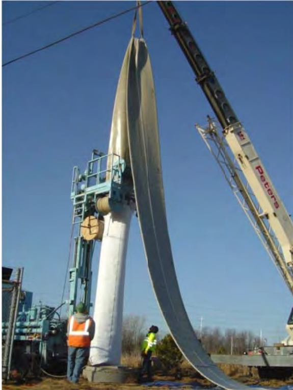
Liner Being Inserted Into Sewer Pipe
