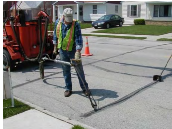
Street Excavation Patch
