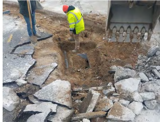
Storm Drain (Catch Basin) Installation
