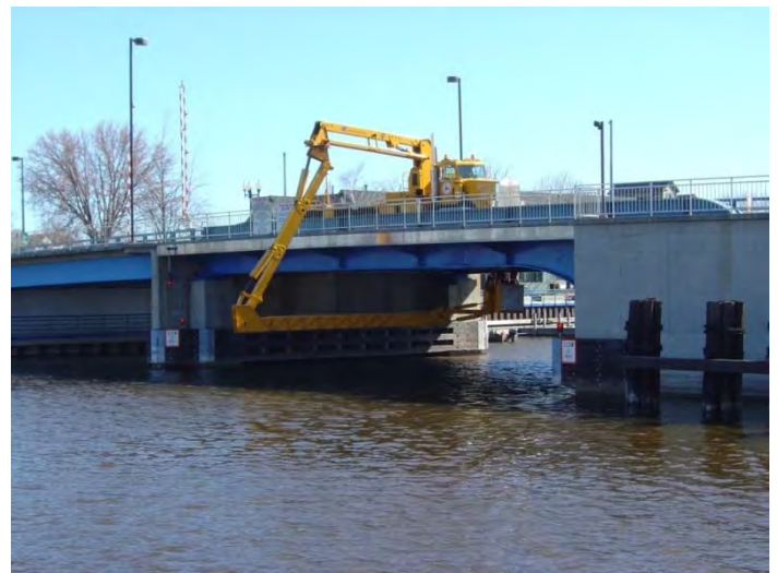
8 th Street Bridge being inspected
