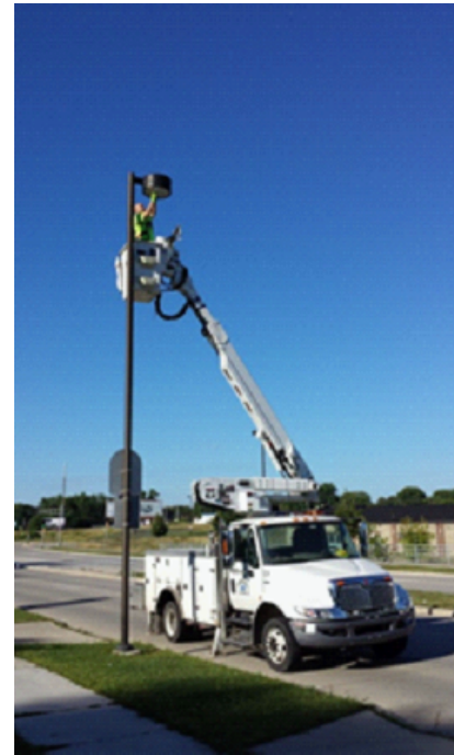
Adding Energy Efficient LED Lighting
