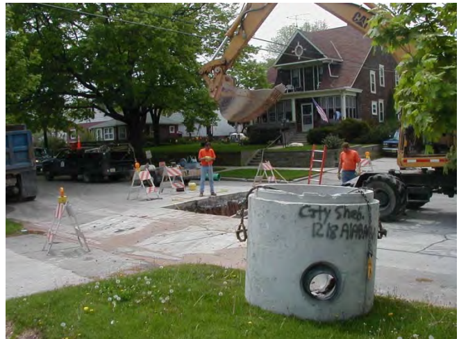
Precast Manhole with Rubber Boot
