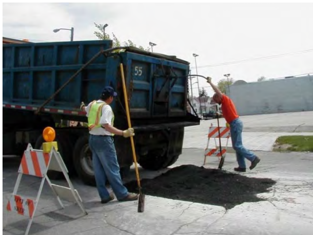
Street Excavation Patch
