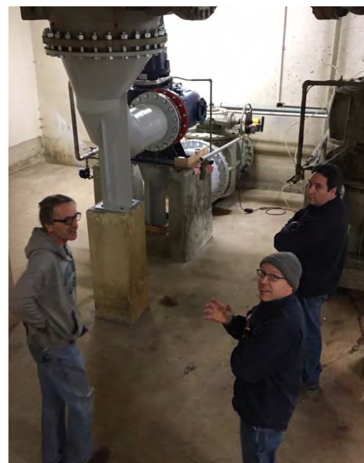
Installation of new Raw Influent Pump
