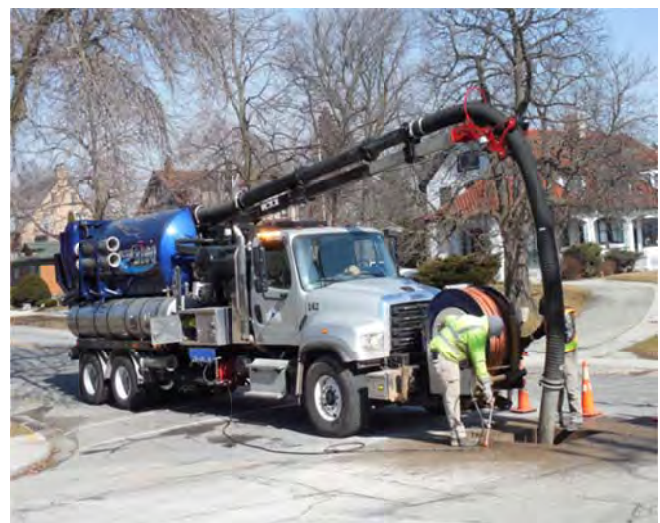
Sewer TV Crew
