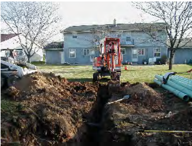
Mini-Storm Sewer Installation - Backyard
