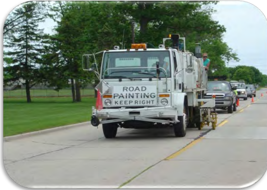
Street Centerline Painting - County Highway Shared Service
