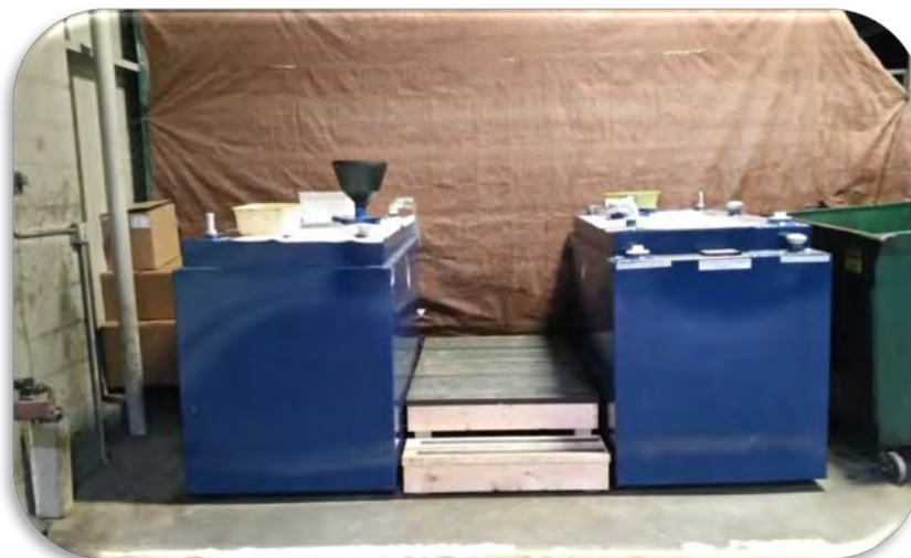
DPW Oil Collection Tanks
