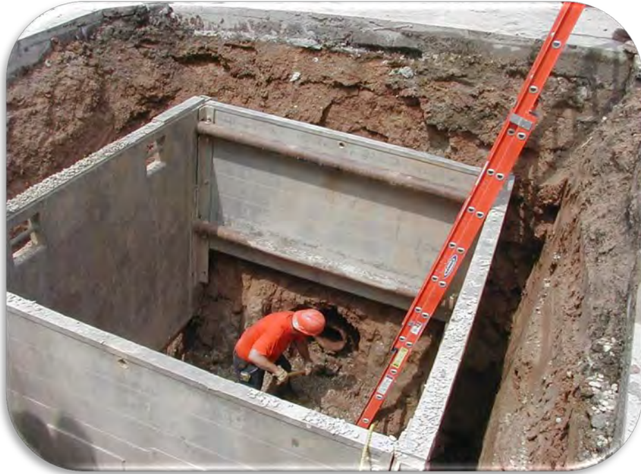
Preparing to Install a New Sanitary Manhole
