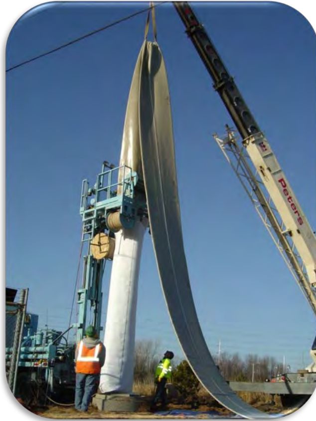
Liner Being Inserted Into Sewer Pipe
