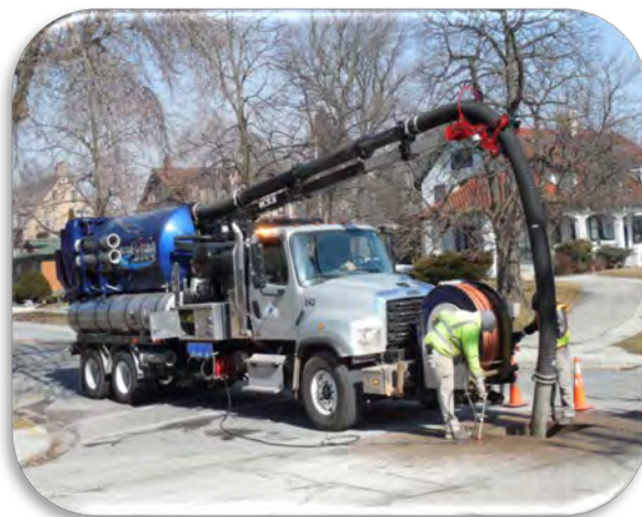
Sewer Vactor Truck
