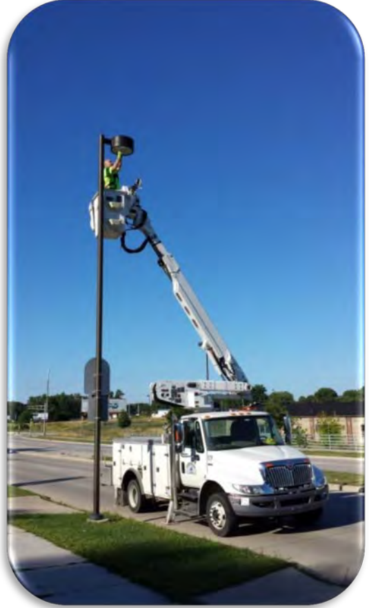
Adding energy efficient LED lighting
