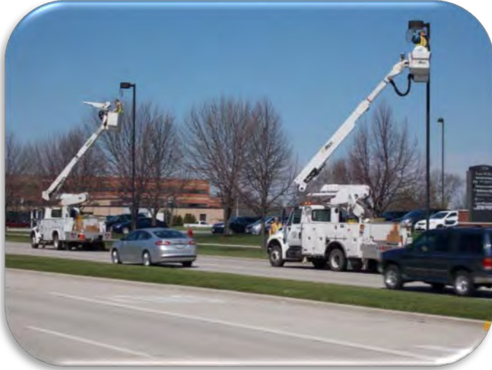
Adding energy efficient LED lighting
