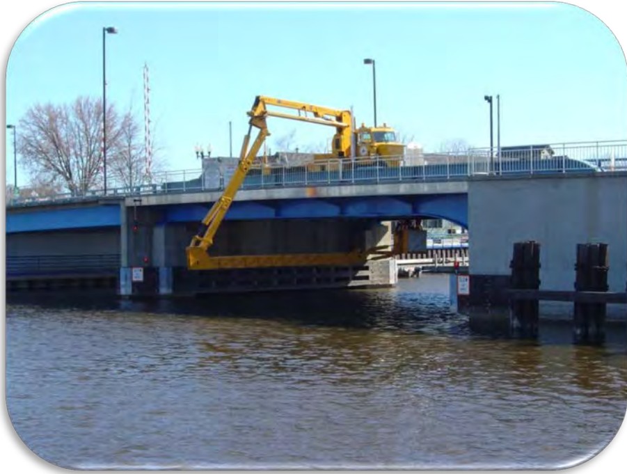
8 th Street Bridge being inspected
