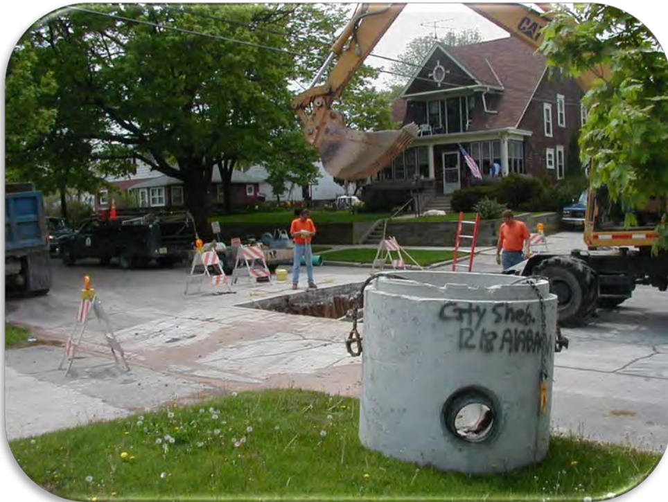
Precast Manhole with Rubber Boot
