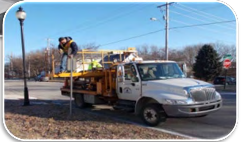
Installation of Signs
