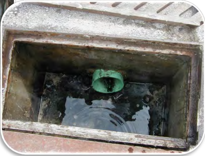
Catch Basin after Cleaning
