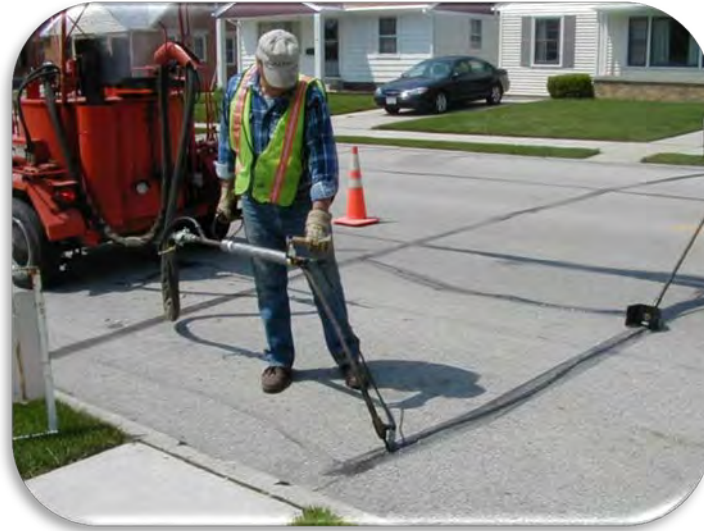
Crack Filling on Asphalt Overlay
