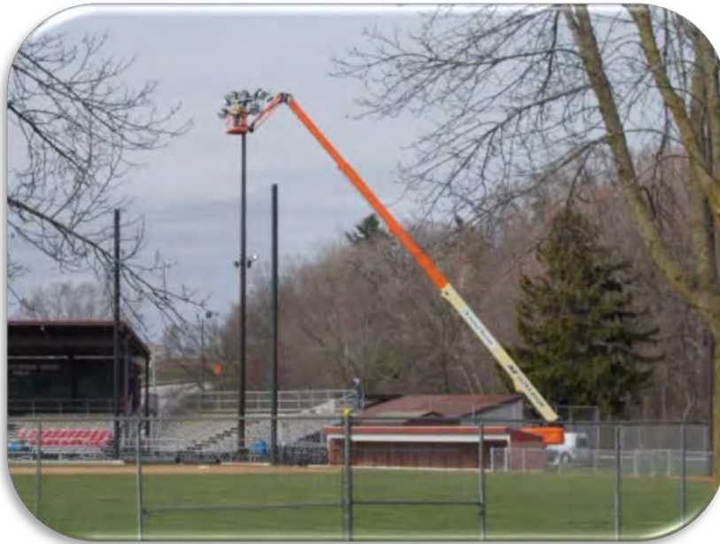
Ball Diamond Lighting Maintenance
