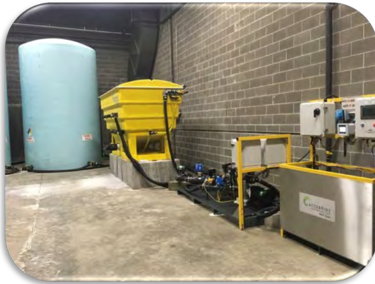
Salt Brine Production Equipment
