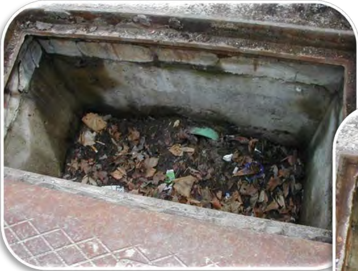
Catch Basin before Cleaning
