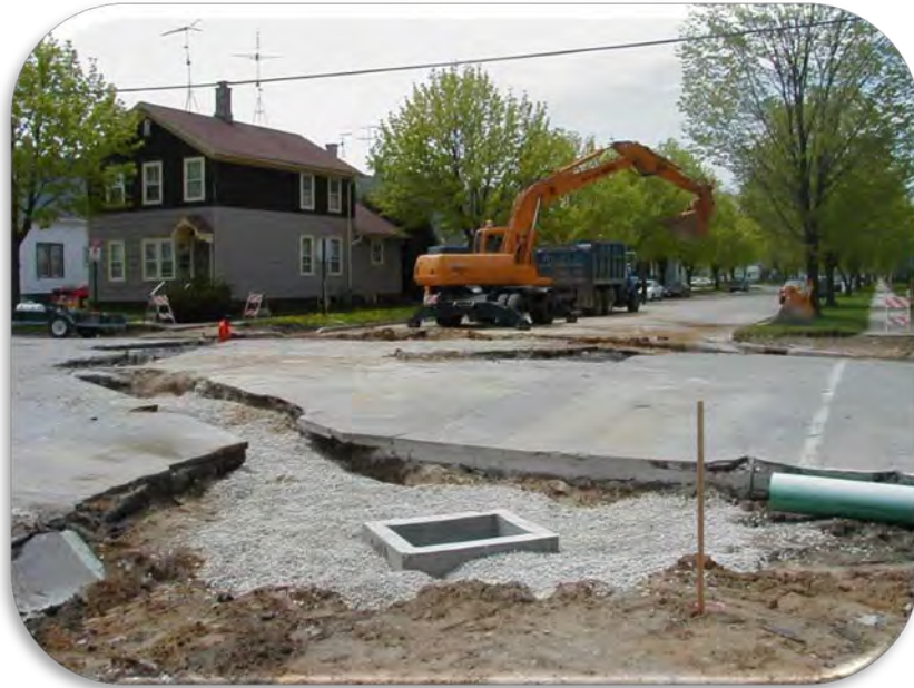
Storm Drain (Catch Basin) Installation
