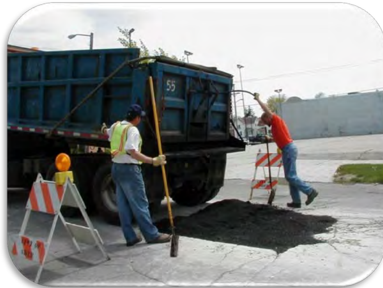
Street Excavation Patch
