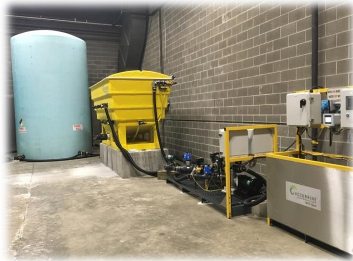
Salt Brine Production Equipment
