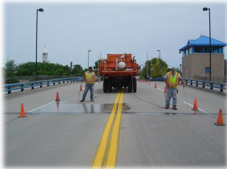
8 th Street Bridge deck being seal coated (County Highway Shared Service)
