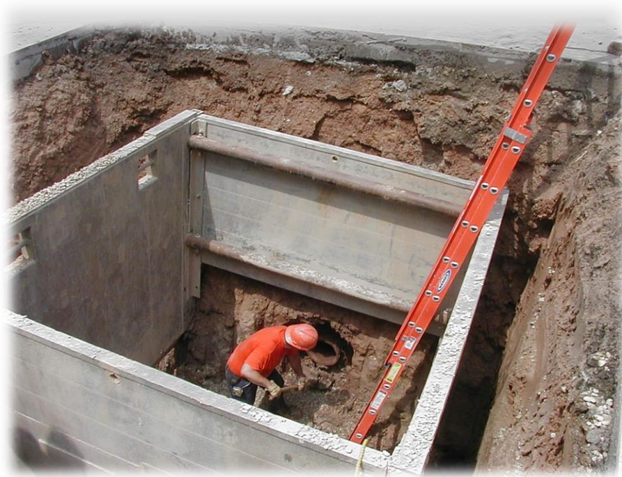
Preparing to Install a New Sanitary Manhole
