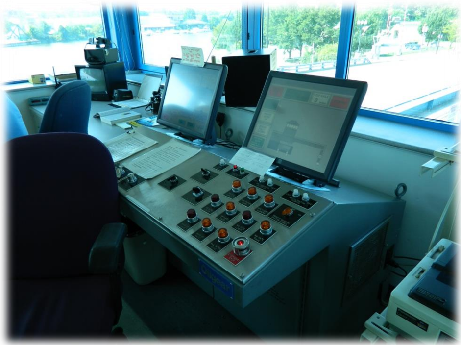
Eighth Street Bridge Controls
