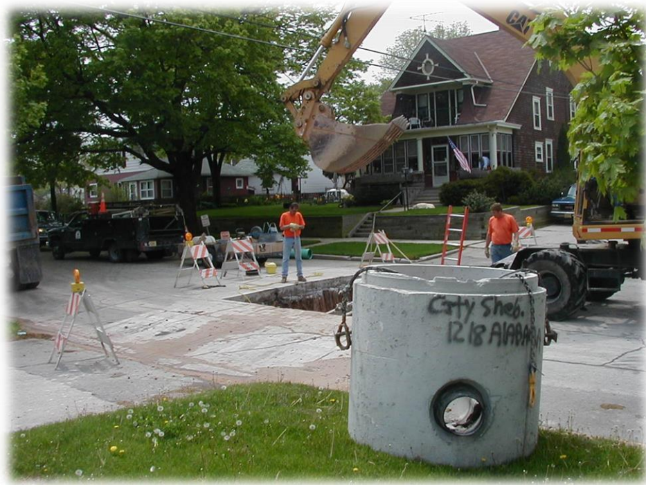
Precast Manhole with Rubber Boot
