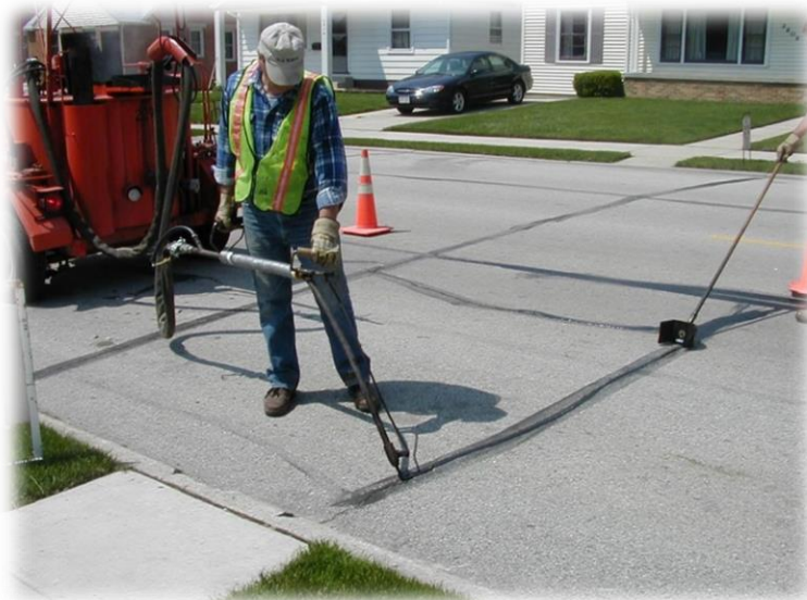
Crack Filling on Asphalt Overlay
