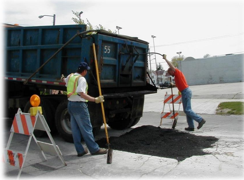
Street Excavation Patch
