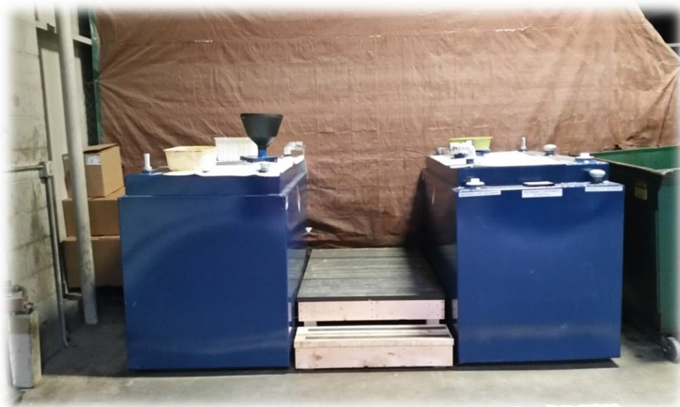
DPW Oil Collection Tanks
