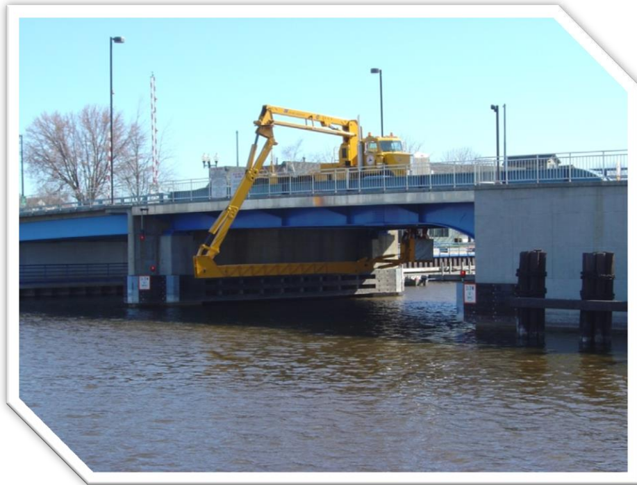
8 th Street Bridge being inspected
