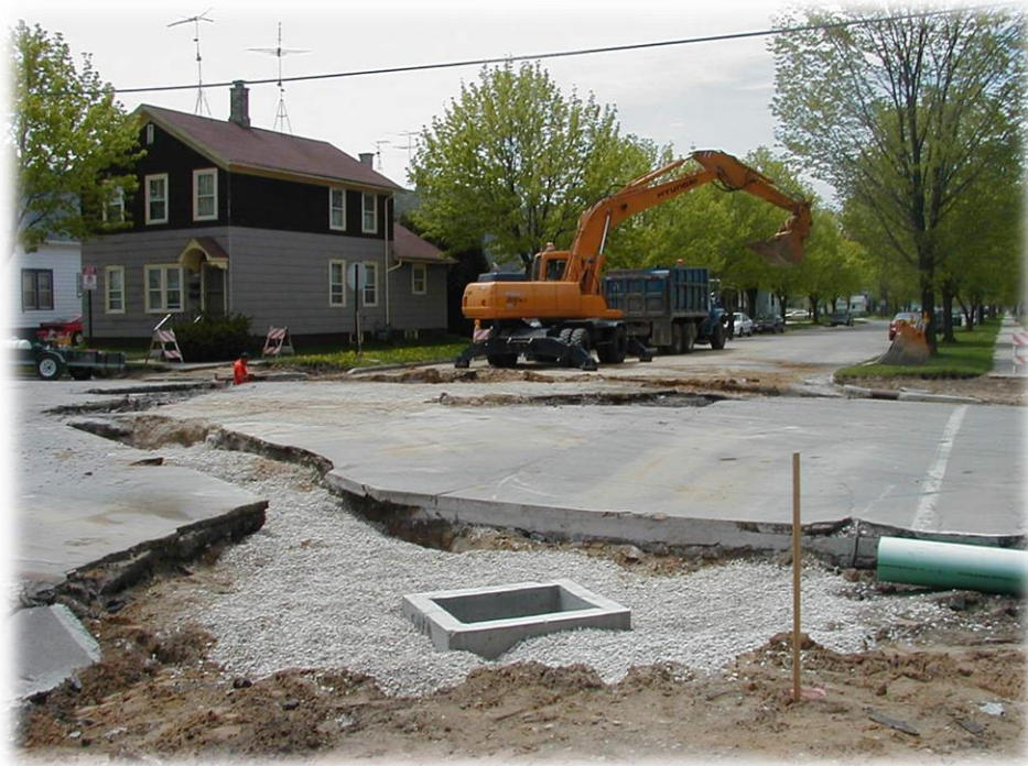
Storm Drain (Catch Basin) Installation
