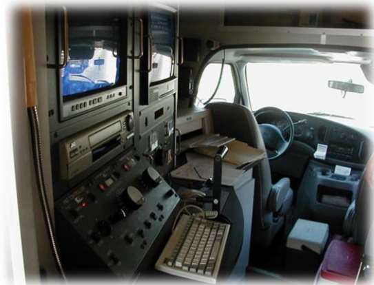
Sewer TV Crew
