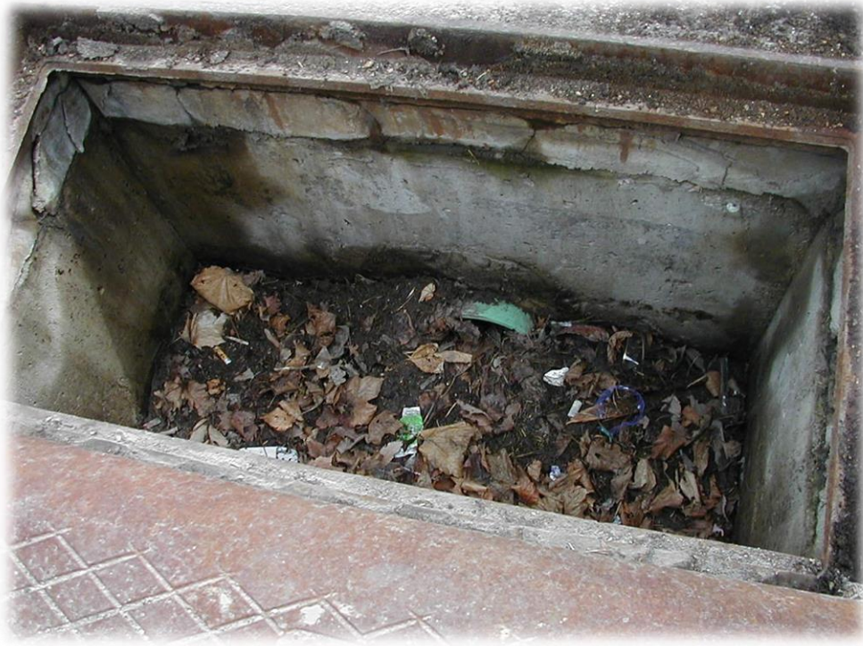
Catch Basin Before Cleaning
