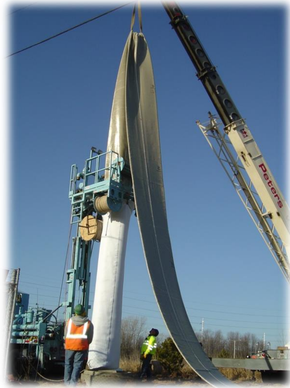
Liner Being Inserted Into Sewer Pipe
