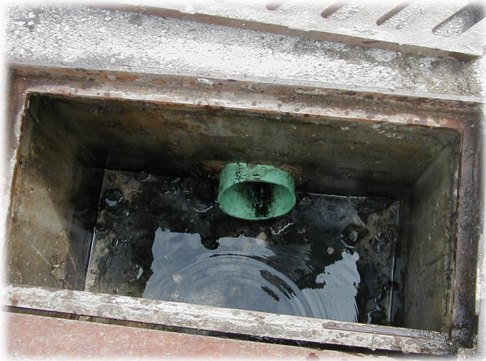
Catch Basin After Cleaning
